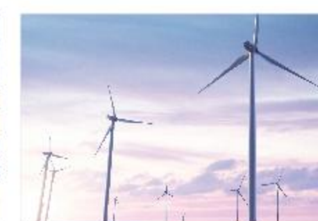
钢铁行业——风机检测
